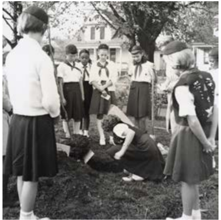
Campfire Girls tree planting at ANIP Information Center, Nov. 3rd 1962. City of Portland Archives and Records A2010-003.2287.
