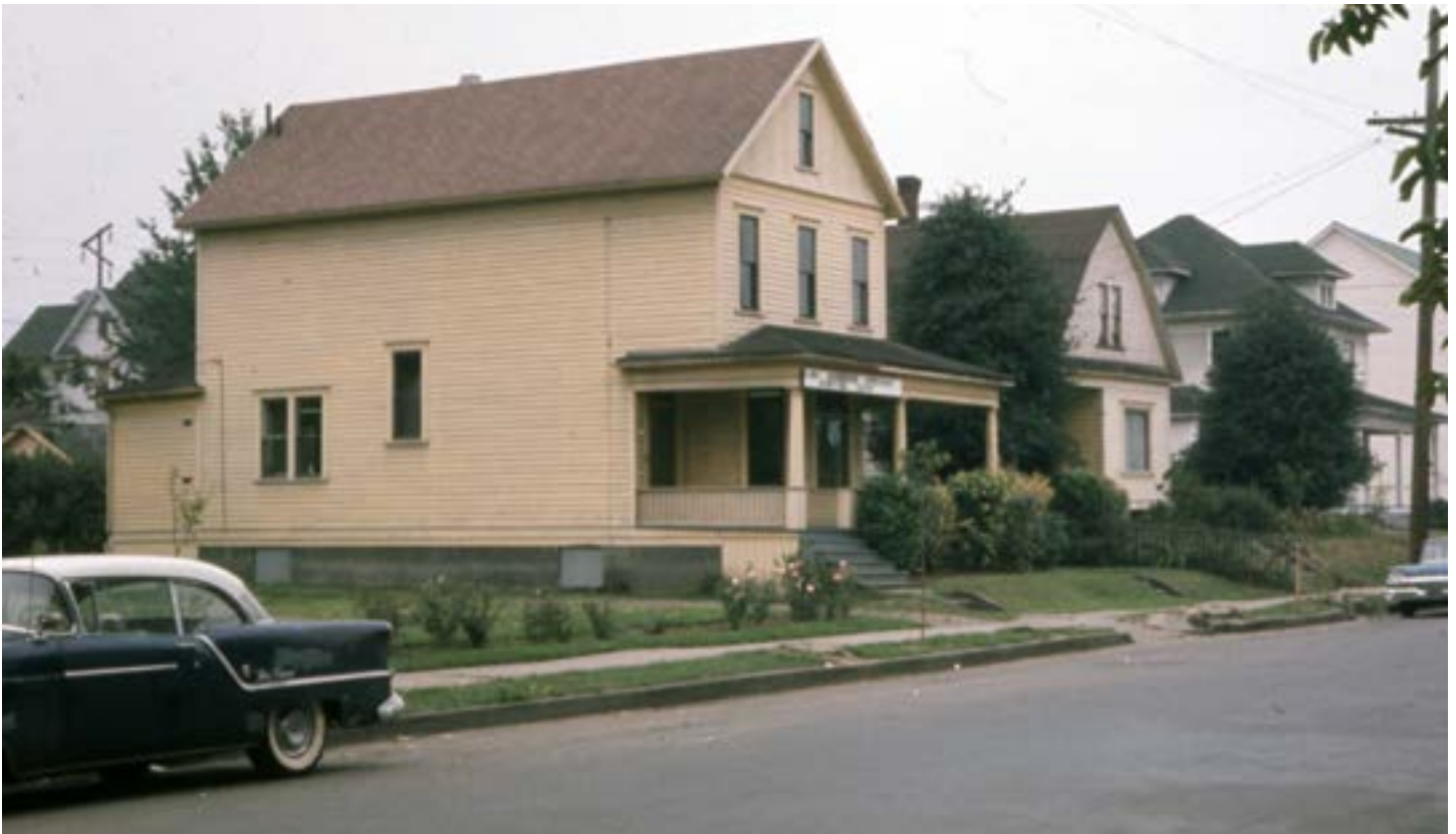
Summer 1963 view of the Albina Neighborhood Improvement Center after tree removals and the replanting of Kwanzan Cherry. The Campfire Girls tree can also be seen over the black sedan. City of Portland Archives, A2010-003.4369.
