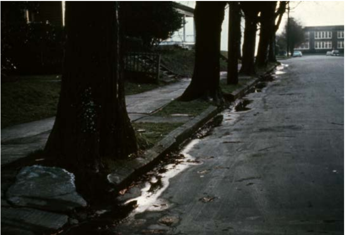
A common sight in 1961 Albina were large trees that were damaging sidewalks and curbs. City of Portland Archives, A2010-003.
